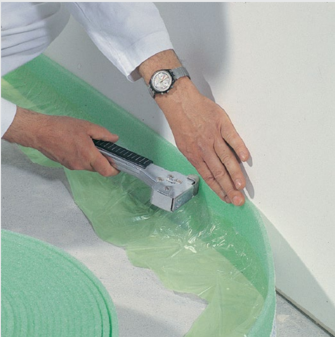
Apply edge insulation strips with foil (also on pipes, radiators, etc.), do not staple at screed height.
