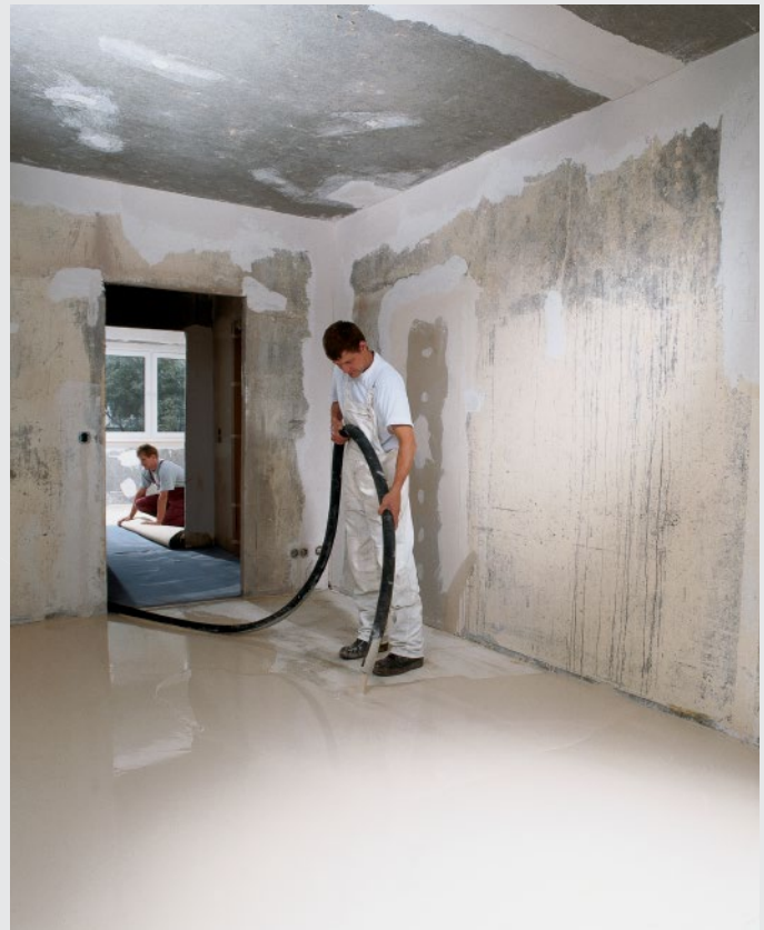
e.g. Machine application of Knauf Nivellierestrich 425
