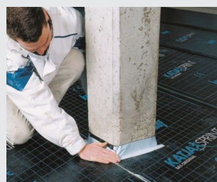
Connections to rising components with Knauf Anschlussstreifen (connector tape)
