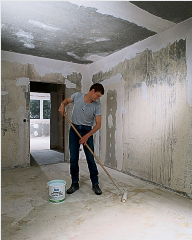
e.g. Prime with screed primer
