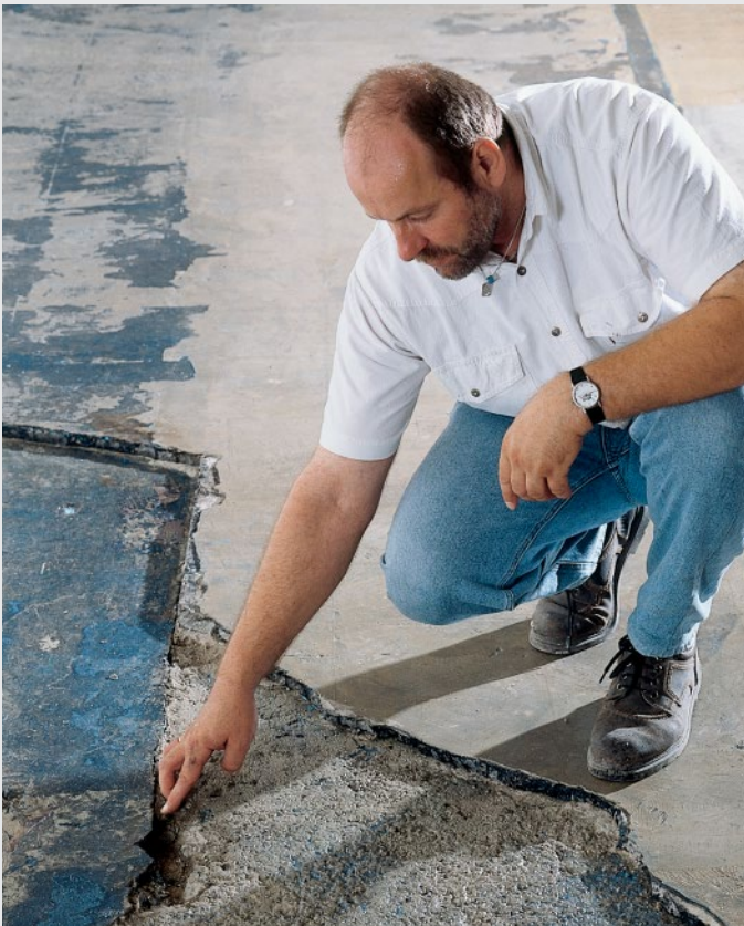
Check the substrate
