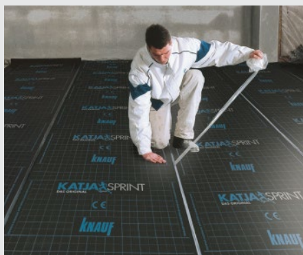
Sealing the long joints by removing the protective film
