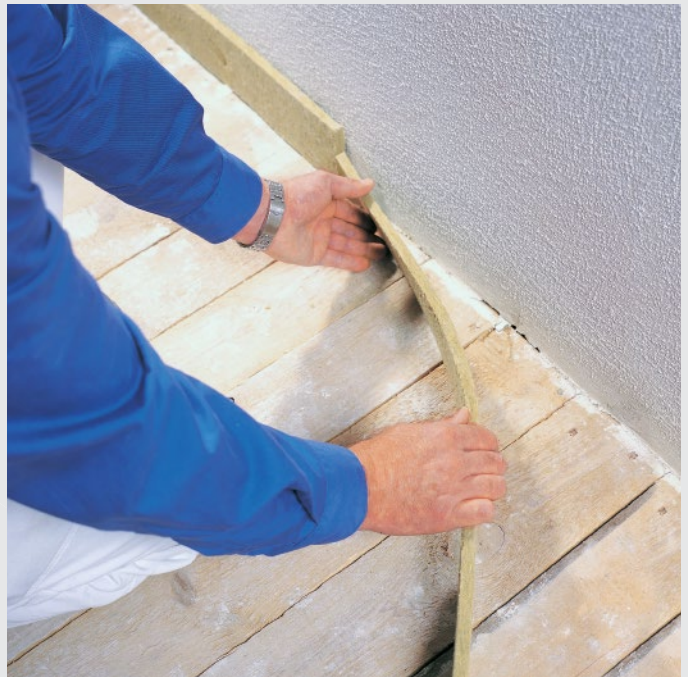
Application of mineral wool edge insulation strips with fire protection requirements
