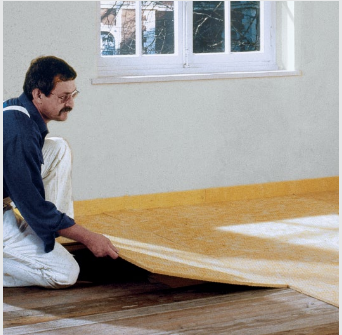
Apply the mineral wool insulation directly against the edge insulation strips and apply row for row
