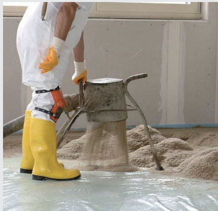
Application with a compressed air conveyor
