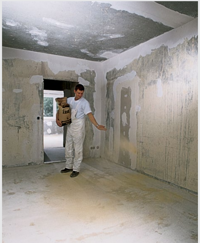
e.g. Bonding primer interspersed with silica sand
