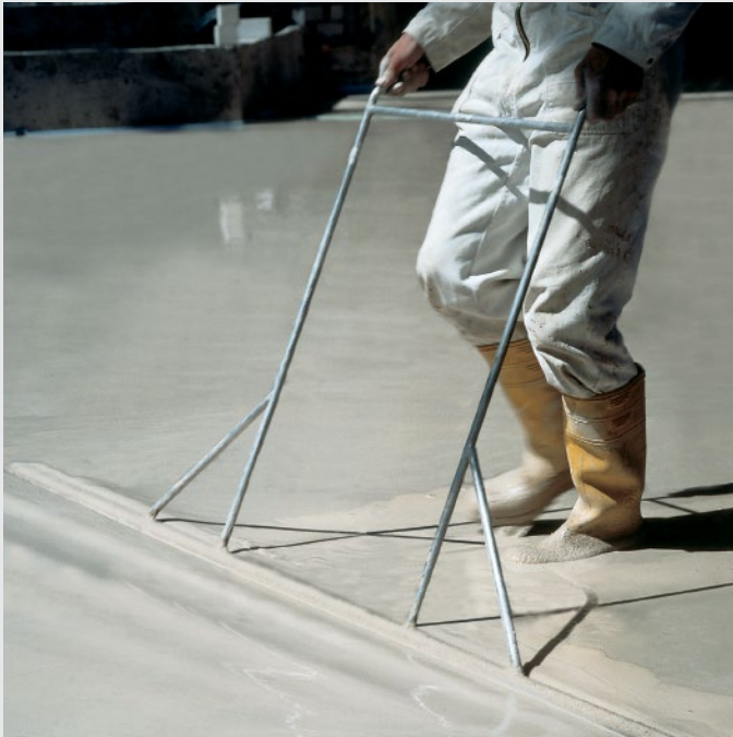
If the screed mortar is to be worked exclusively with a dappling bar after application, the lower slump flow value should be aspired to.
