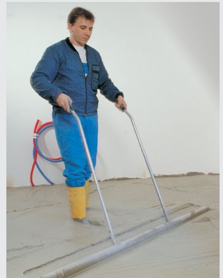
After material application simply level with the dapping bar
