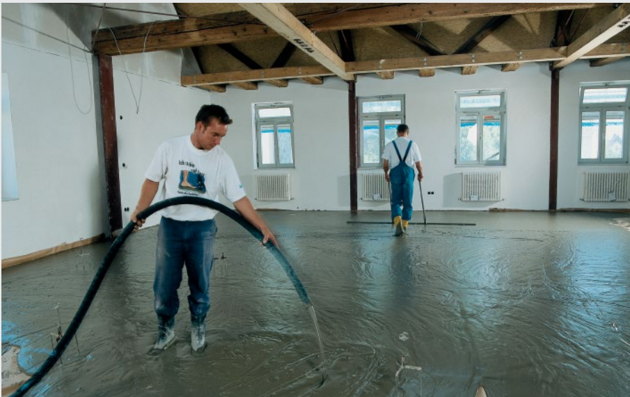
Knauf Schubo now flows and seals cavities where previously polystyrene was cut and applied meticulously
