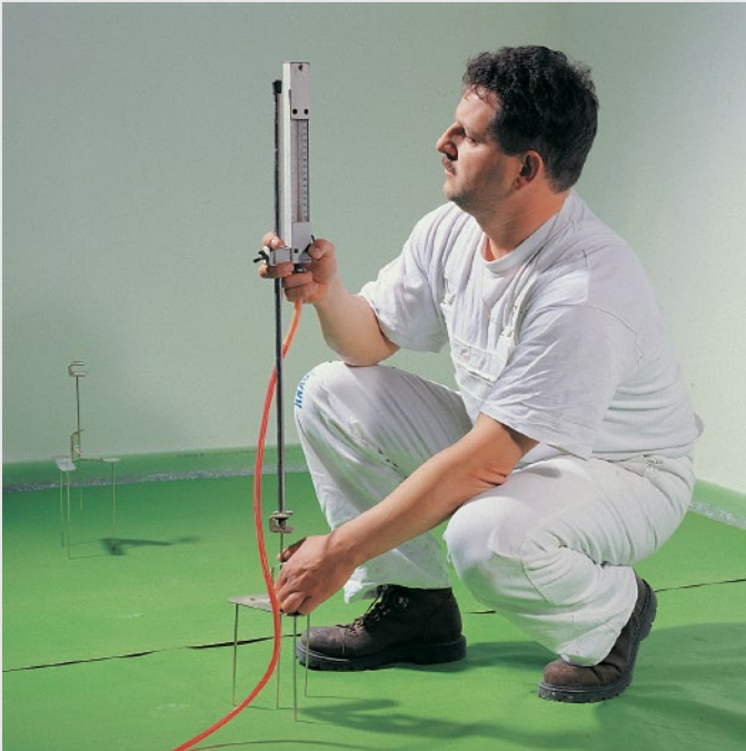
Setting the height with PFT Levelling Sensors
