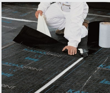
Sealing of front end joints with Knauf Anschlussstreifen (connector tape)
