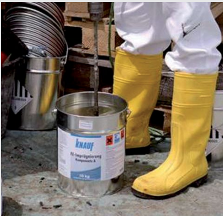
Mixing of the epoxy resin with a mixer
