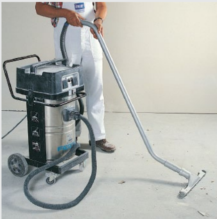
Cleaning with an industrial vacuum cleaner
