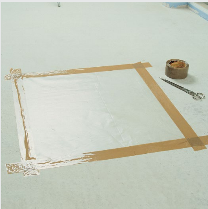
Initial inspection of drying with foil on the heating floor screed
