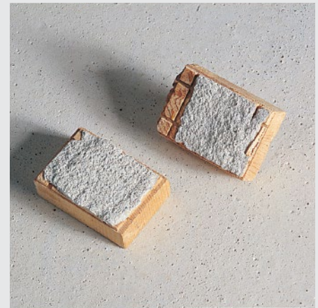
Parquet and screed failure patterns
