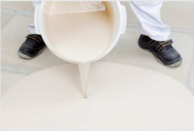
Filling of the screed with Knauf Nivellierspachtel 415
